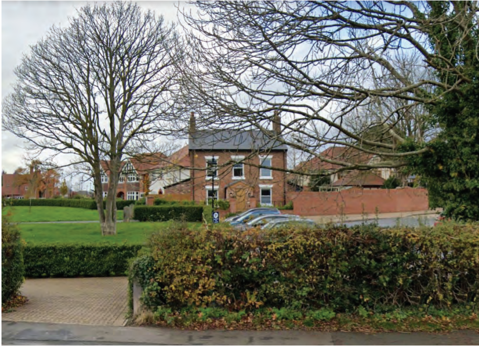
Tucked away now, behind the car park in the village centre, restored, loved and looked after again, the Grange Farm house has had a new lease of life.
